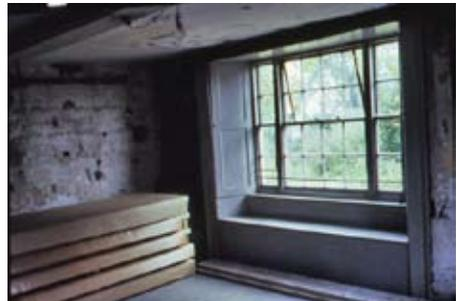
room an ingenious series of pulleys were slowly and gently pulling the damaged wallpaper off to be laid in boxes for restoration, the same process was being carried out in the garden room. The bare walls were in a sorry state, the plaster crumbling, large holes pierced the ceilings and damp places splattered the walls.
